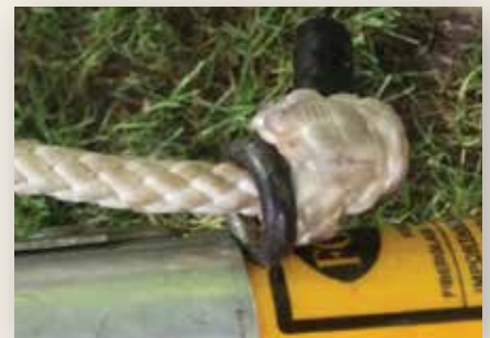
Hole has been drilled in pole and an attachment added. This is an UNACCEPTABLE PRACTICE!
